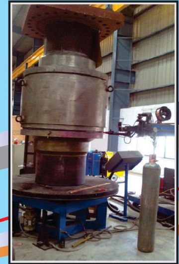
BALL VALVE ROOT TIG WELDING SYSTEM
